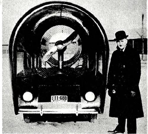
Constructed as a demonstration model for government officials this strange automobile pictured here with its inventor, Thomas Finley, is driven by a propeller revolving in a wind tunnel.
