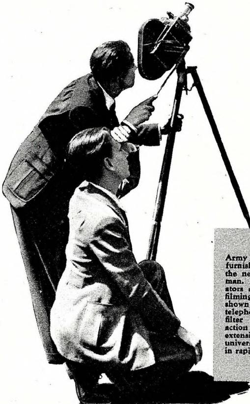
Army air maneuvers furnish a real test for the newsreel cameraman. Here two operators are engaged in filming the planes shown above using a telephoto lens and filter to bring the action closer. A long extension arm and universal tripod aid in rapid follow shots.
